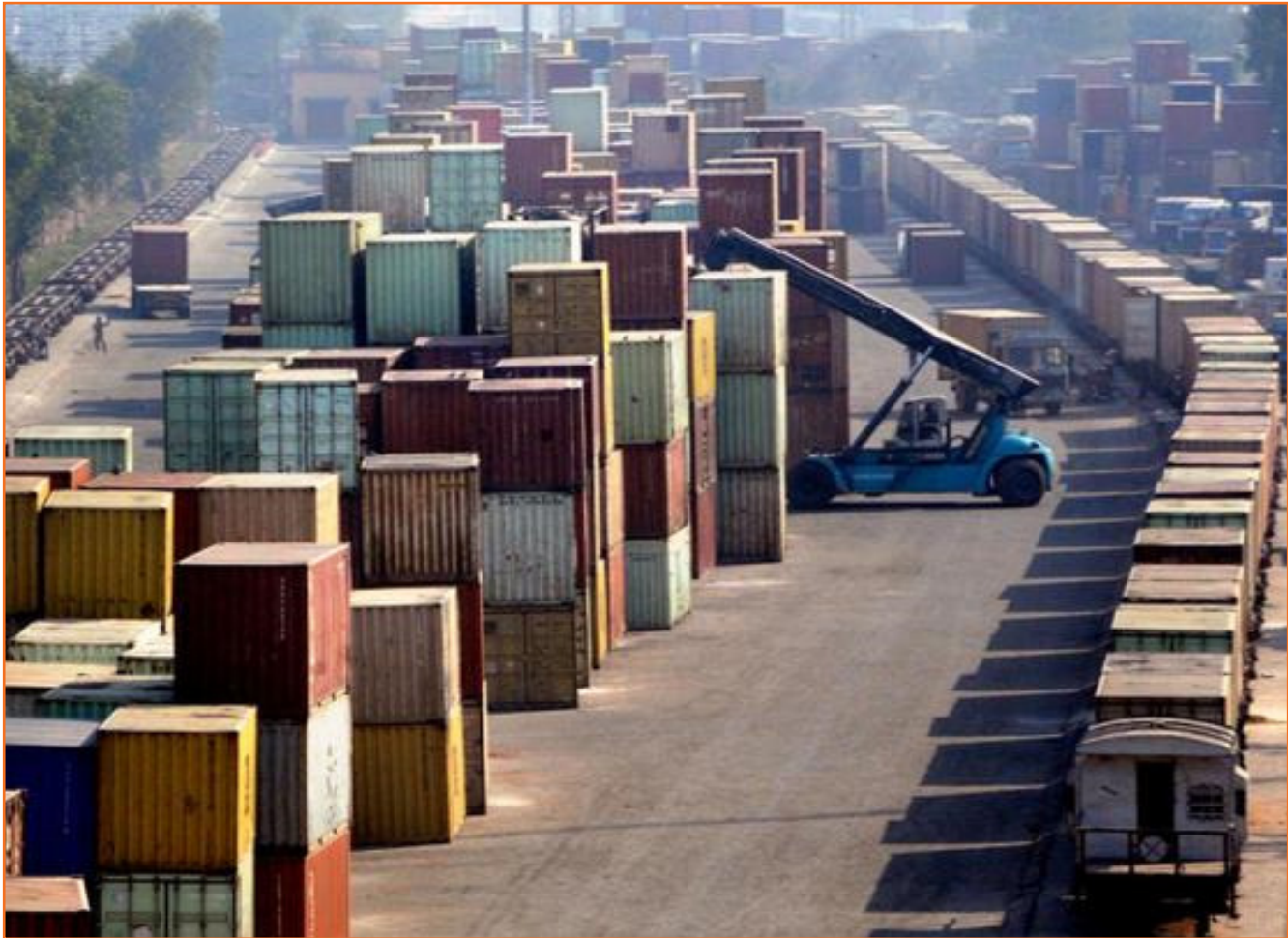
Fig.5.1.11: Inland Container Depot
